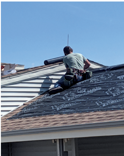
A volunteer helps with repairs after the derecho.
